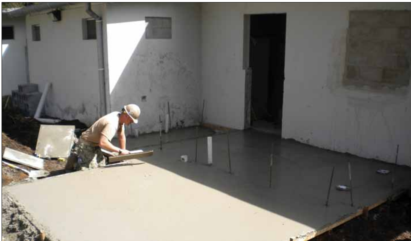
▲ Utilitiesman 1st Class Andrew Duquette, assigned to Navy Mobile Construction Battalion 27, performs finish work on a concrete slab at a Guatemalan military base. U.S. Navy photo by Lt. j.g. Keith Ferreira.
