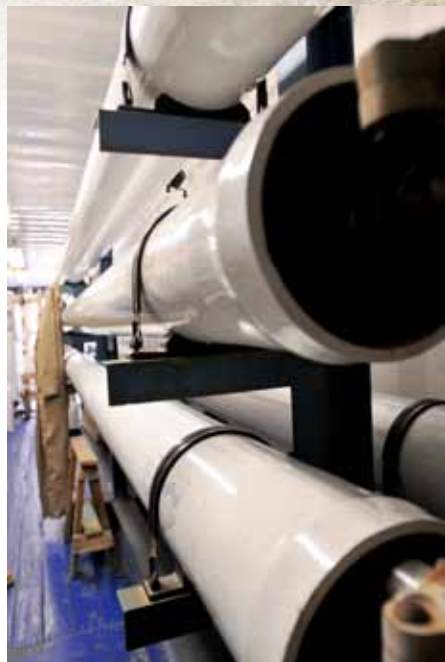
Water passes through these tubes, which are filled with membranes designed to remove particulate matter, as part of the reverse osmosis process.
