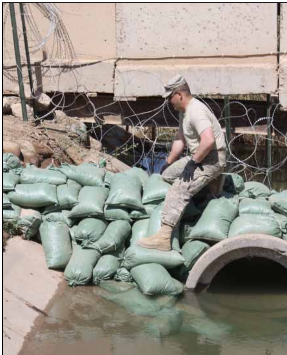
Staff Sgt. Brad Wilson, from Sandusky, Ohio, a member of 1192nd Engineer Company, places a sandbag on top of a culvert at Victory Base Complex March 19.
