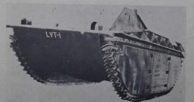
LVT-1, 1941-1943 Engine: Hercules, 6 Cyl., 150 hp Speed: Land, 12 mph Water, 6.1 mph Cruising range: Land, 150 miles Water, 60 miles
