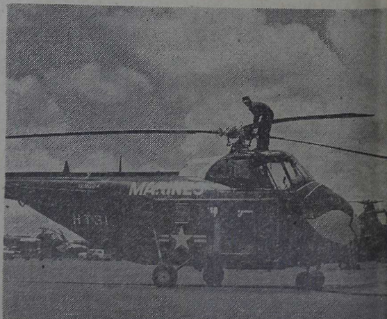
SECURE THE DETAIL —Cpl. William Smith begins the securing of the detail after flight by letting the blades down and hinging them to the side.
