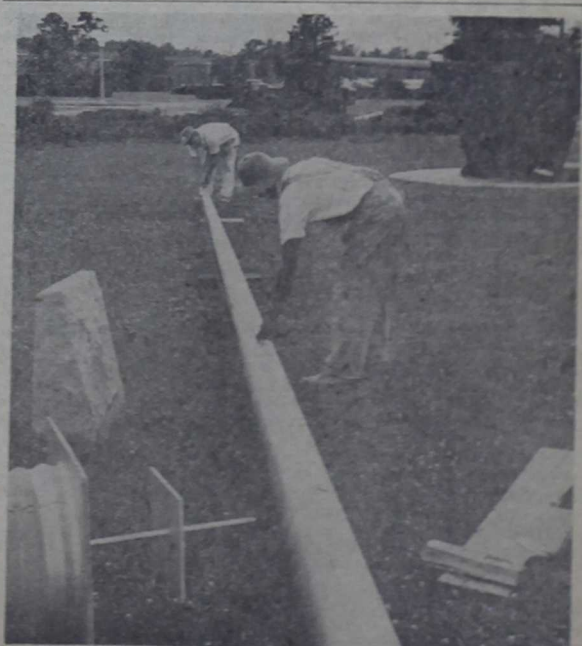
LONG MEASURE —Workmen from Camp Maintenance take the measure of the 76-foot flagpole to be placed in front of Bldg. 1. Before the pole could be positioned, workers had to drill through about seven feet of concrete to sink a foundation. The job began Monday and is expected to be completed today.
