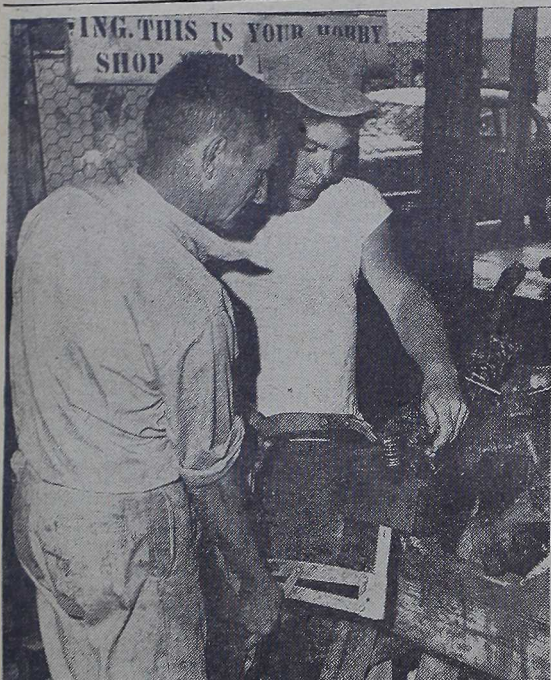
VALVE REMOVER —Arnie Aman, left, chief mechanic in the auto section, shows Pfc Charles D. Jones, 4.2 Mortar Co., Second Marines, the correct method of removing the valves from his engine.
