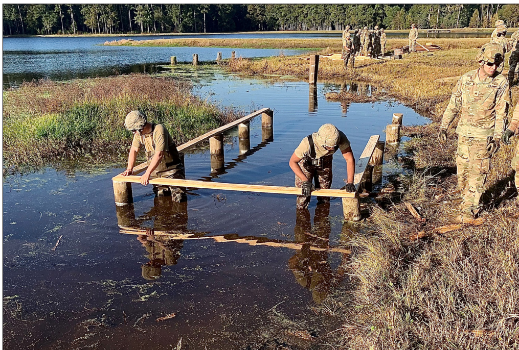
Soldiers installing the base of the wharf superstructure onto the piles.
