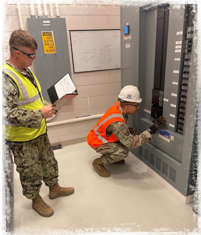
Service members review and analyze single-line diagrams in conjunction with circuit breakers.
