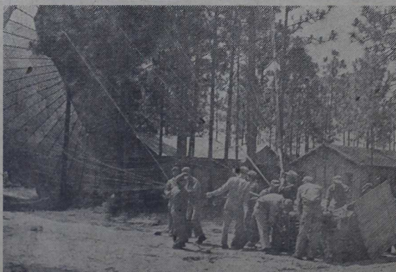
MODERN GUNGA DIN—That's the story of these members of the 2nd Engineer Bn. who work as a team to provide water for thirsty Leathernecks. Equipment for the purification of water is dropped from an R4Q "flying boxcar" and in a matter of minutes a "water point" is erected, where in one and a half hours enough water for a regiment can be purified (Official USMC Photo).
