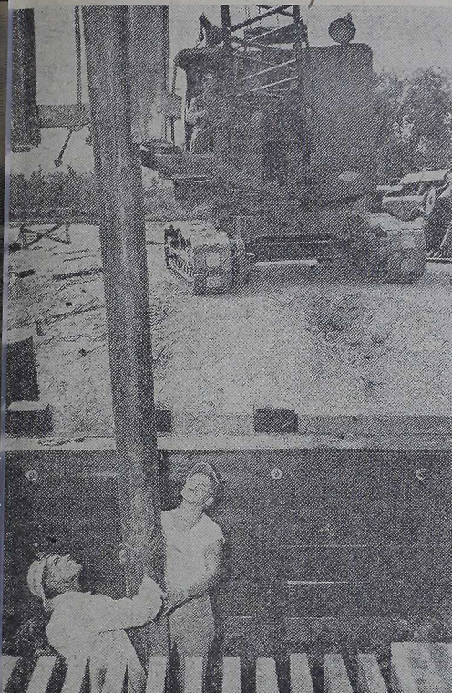
BRIDGE PILE hits bottom of Scales Creek between Camp Knox and Fort Point as the 2nd Engineer Battalion's new bridging units get underway. Forty men are building the 190-foot bridge under the guidance of 2nd Lieutenants R. H. Van Meter and Stephen Lin. Twenty feet wide, it will carry approximately 100 tons (Official USMC Photo).
