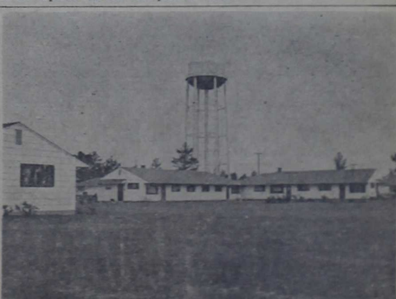
TERRACE TANK—Simultaneous completion of the filter plant's new 250,000-gallon elevated tank and the last few housing units of Tarawa Terrace II brings the dwelling facilities of the two "Ter- races" to 2,108 family units. They have a water consumption capacity of 1,000,000 gallons daily (Official USMC Photo).
