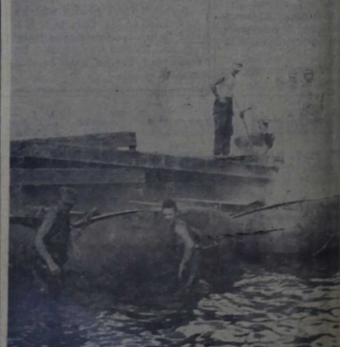
WET WORK—Waders attach towing lines to two bridge sections. Men of the Bridge Platoon, secure the sections together prior to moving them into position. The "fog" which covers the area was produced by the 1st Provisional Smoke Platoon, which journeyed from Camp Geiger to Montford Point last Wednesday to participate in the exercise (Official USMC Photo by Cpl. Don W. Sharpe).
