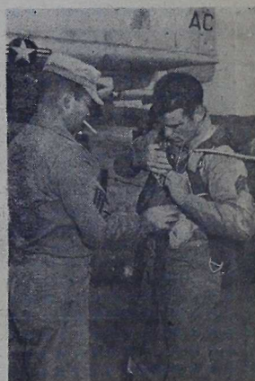
THE EMERGENCY CHUTE is a vital part of the jump gear carried by each parachutist—just in case the back pack fails. Here Sgt. Jack Stodghill, right, gets a hand in adjusting his harness to take the smaller safety chute from TSgt. Robert Chose . . .
