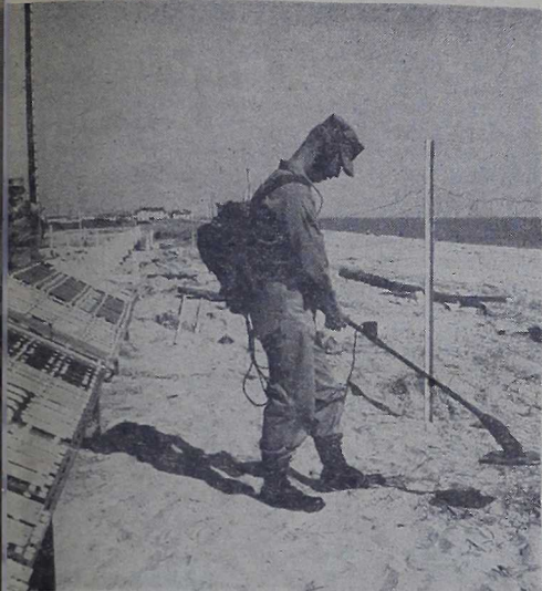
RPS TREASURE HUNT—Sgt. William E. Dilsaver, right, Clinton R. McCarthy make with the mine detectors in -times search for buried treasure as they sweep for specimens lost in the sand at Kure Beach. Part of a sea osion experiment underway since 1935, 1,500 metal plates ed by Hurricane Hazel last month. The team found more ) of the lost plates (Official USMC Photo).
