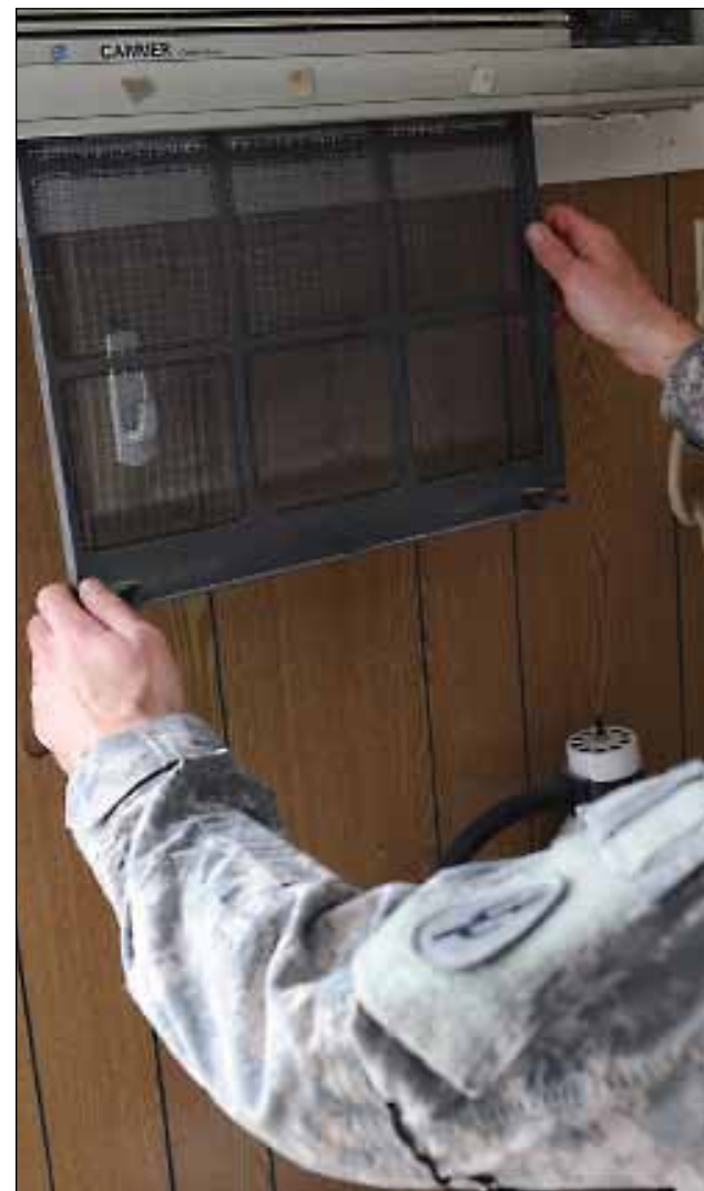
Pull the filter from an air conditioner in order to clean it. KBR officials warn against spraying air freshener into A/C units because they are oil-based and will cause dirt to stick to the filters.
