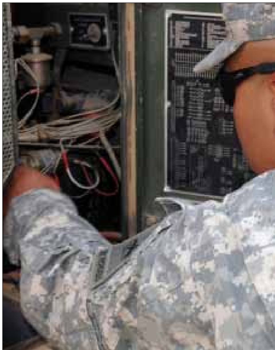
Spc. Jose Barrera, a generator mechanic, examines the wiring of a non-functional generator while troubleshooting what is keeping it from starting.
