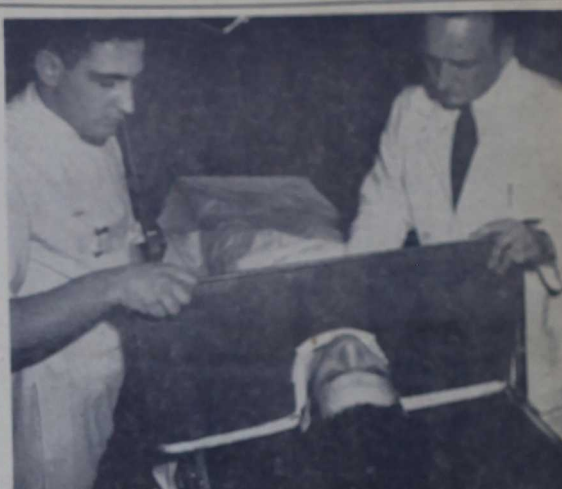
IDEA IN ACTION —The idea's effector, HM3 Francis Perrelly, left, and the idea's originator, LT Frederick R. Latimer (MC-USN), right, demonstrate their home-made arteriographic shield, designed to protect X-ray technicians from radiation (Official USMC Photo).
