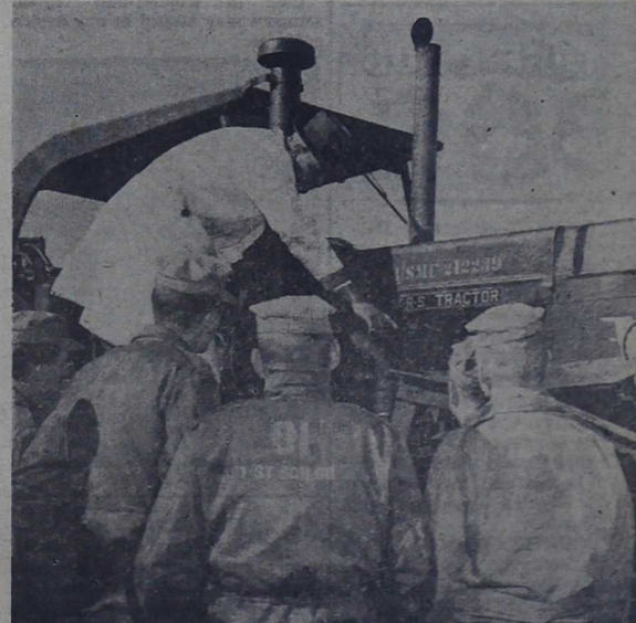
TROUBLE SHOOTING —Leonard Young, a sales representative for Cummings Diesel Co., explains to a class in the Engine Equipment Mechanics Foreman course the operation and maintenance of his product. For four days the class studied the adaptability of the 300 HP diesel engine in a Mississippi Road Service tractor.
