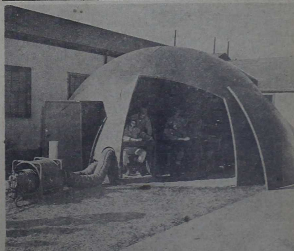
HOME-ICILE!—Marines of the 8th Communication Bn., Force Troops, are shown testing new communication equipment at Camp Elmore, Norfolk, Va. When completely assembled the hut forms a perfect hemisphere. Apparatus at far left is the heating and air conditioning unit.
