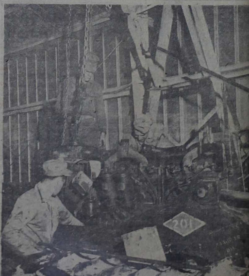
FINISHING TOUCH —Members of the Heavy Equipment Plt., Co., 2nd Shore Party Bn., responsible for repair of heavy equipment such as cranes and tractors, make final adjustments after installing radiator in a landing force tractor, used to tow mired vehicles amphibious landings. Laboring are Sgt. Tony Drapak, left, Cpl. L. Ball, standing, and Cpl. Stanley W. Taikowski (Photo by Pfc Maurice Blier).
