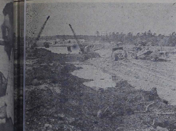
Construction proceeds on two additional lanes for Highway 17 along a five-and-a-half mile strip between the Main Gate and Sonville. Widening of the road began February 21 and lanes are expected to be ready for traffic by late September or early October. Cost of the project is divided between state, federal government from highway appropriations, and "military money" voted by Congress to provide better roads into military installations.
