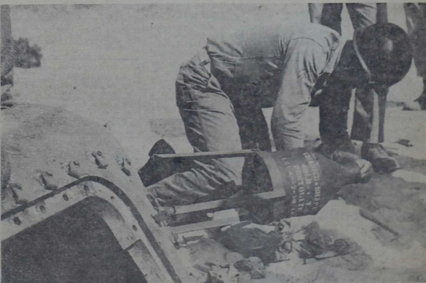
A SHAPED CHARGE is placed on a tank turret by Cpl. E. R. White, assistant instructor. The explosive charge will penetrate the heavy steel armor and greatly damage the inside parts of the turret. . .
