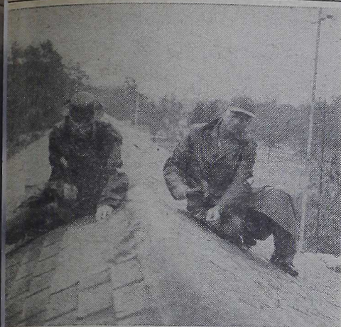
WINDS BLEW —Fast as Hurricane Diane blew 'em off, Camp Maintenance carpenters nailed the shingles back of Capt. V. B. Haws' quarters at Paradise Point during of the storm Wednesday. Secure in their rooftop perch P. Cole, left, and Charlie H. Pulley, part of a standby maintenance men that went from roof to roof in an effort more serious damage (Photo by Sgt. Emil Dansker).
