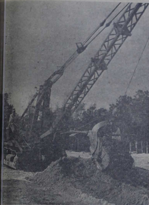
AT SCOOP work with this dragline crane, mounted on a "cat" tractor, means Pfc N. C. Hope has learned to operate tricky problem in the Equipment class.
