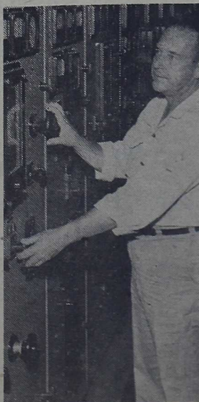
POWER PLANT—Samuel S. Holland, Dispatcher at Lejeune's Electric Generating plant on Highway 24, is synchronizing the Fairbanks-Morse Diesel generator with the Lejeune-Cherry Point power system to enable both reservations to have electricity.
