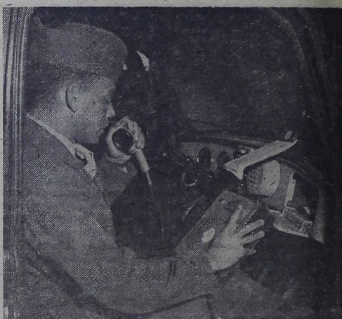
TIMING ALL CARS —Sgt. Albert Jones, Headquarters Company, and Traffic Investigator for the Provost Marshal, is operating electric timing device called the "Whammy," and calling another patrol car to catch speeding violators on Lejeune's main gate.
