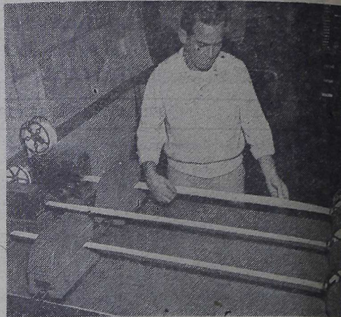
HOT NEWS —Bobby Adams, one of three dispatchers for Camp Fire Department, is taking a reading from tape on the Acme Fire Alarm System which furnishes information pertaining to the local fire at Camp Lejeune. This instrument is hooked up to more than 300 alarm boxes around the base.
