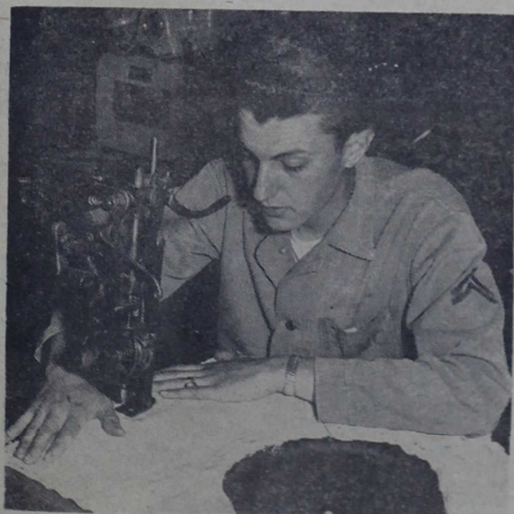
START OF A VEST —Cpl. Stempowski sews layers of basket weave nylon together in initial production stage of anti-fragmentation tropical vest.
