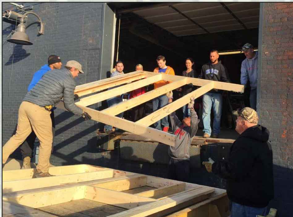
The team pitches in to load a wall frame constructed at the Habitat for Humanity workshop for transport to the construction site.
