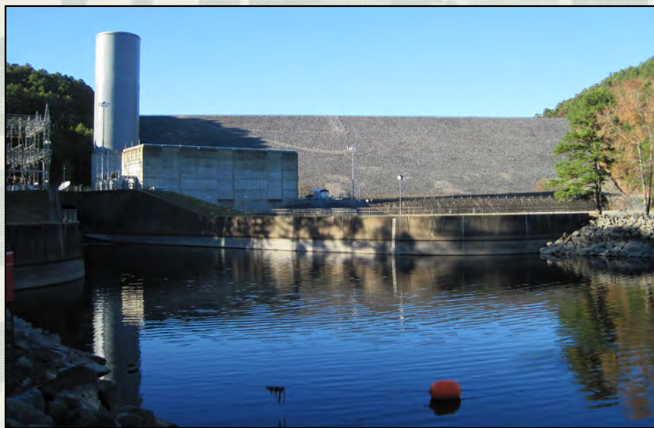
The LRL Risk Cadre team performs a site reconnaissance meeting for Blakely Mountain Dam, Royal, Arkansas. The project consists of a 231-foot-high earthen embankment dam with a hydropower power plant located in lower left of photo.
