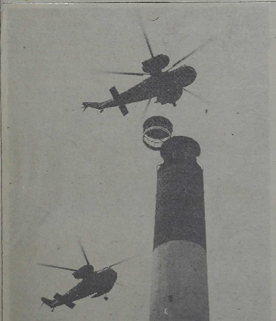
UNIQUE AIRLIFT —One Marine helicopter from MAG-26 lifts into place a 1,740-pound lantern atop the Coast Guard lighthouse at Oak Island, N. C., as another stands by as observer and control for the operation. The 20-million candlepower lamp which was installed recently will make the new lighthouse the most powerful on the East Coast with a range of up to 24 miles.
