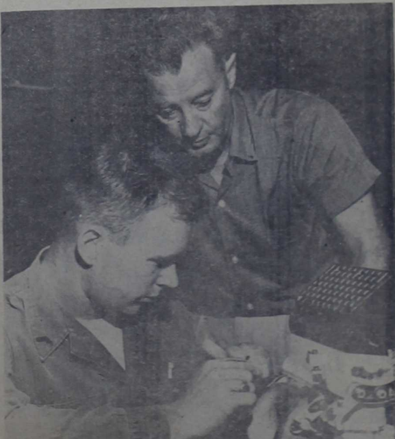
PRECISION WORKMANSHIP —Fire control and optical instrument instructor Charles T. Hill watches closely as Corporal John L. Puls delicately adjusts the periscope on an eight inch self propelled howitzer.
