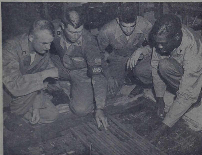
THE BIG ONE WORKS THE SAME WAY —MSgt. Mile J. Tyler demonstrates on a model of the M4T6 floating bridge the proper way to assemble it before Cpl. David H. Montague, left, Pfc Jack
