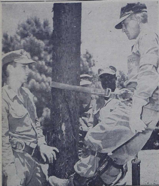
KEEP THAT LEG STIFF —Pfc. Ronald J. Lewis, left, Pvt. Don B. Reier, and Sgt. John H. Holmes of the 1st Engineer Bn., are reviewed on the important points of pole climbing by TSgt. Dewey J. Wilburn in the Basic Electricians Class.
