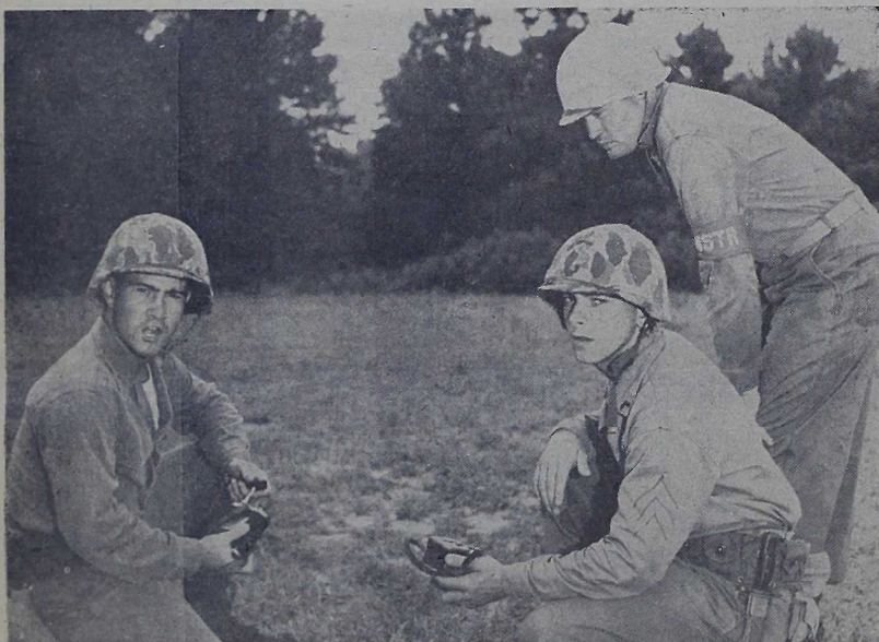
FIRE IN THE HOLE —Cpl. Richard A. Derbert, USMCR, gets ready to set off a charge of TNT as Cpl. Robert J. Anuszewski, USMCR, makes a last-minute check of the circuit with a galvanometer.
