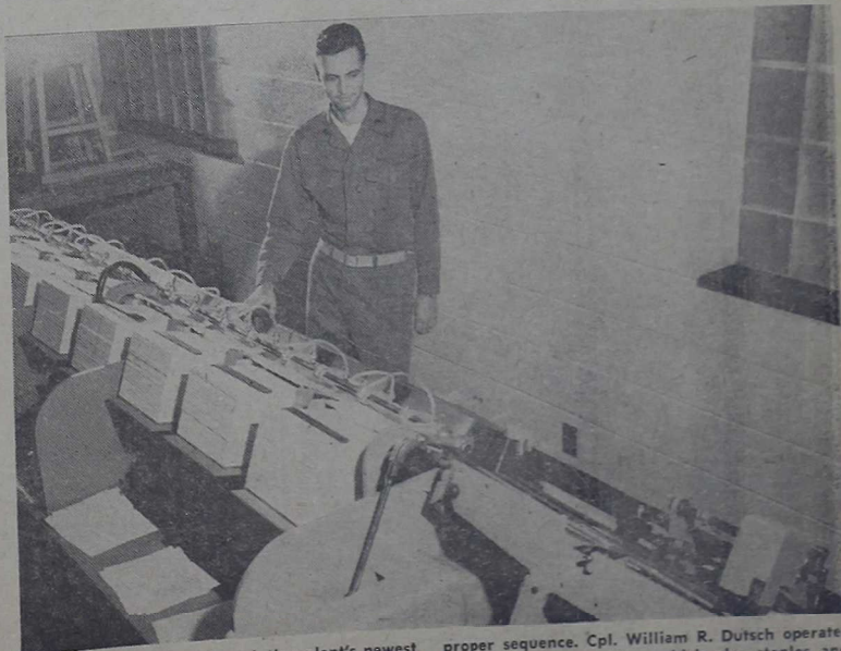
ARRANGING PAGES —The printing plant's newest machine is this collator which arranges the pages of books, pamphlets and other material in their
