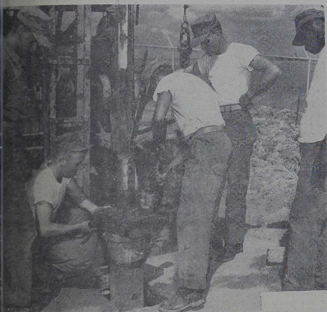
DAY BREAK —Finds the Eighth Engineers operating the percussion drill used to dig wells. The five-man crew, headed by TSgt. James Fischer, gets ready to put in a new cast. All hands are required to attach each 10-foot section cast.
