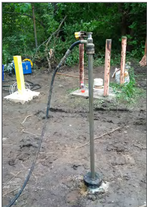
Field work at Nike C-47 included injecting sodium lactate into the groundwater to reduce TCE levels.
