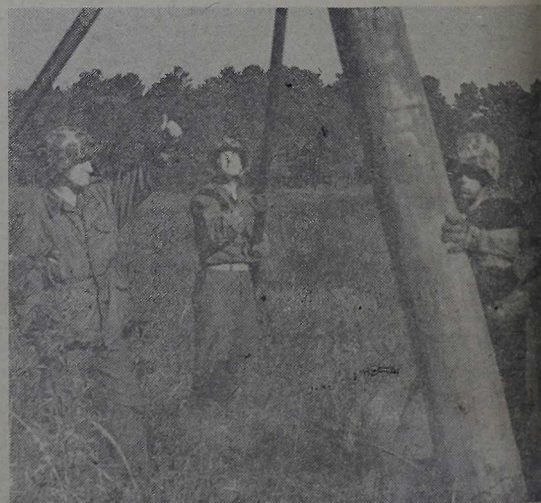
NEARING COMPLETION —Pole is edged into place with the aid of supports. After the pole is positioned, dirt is packed around its base to secure it.
