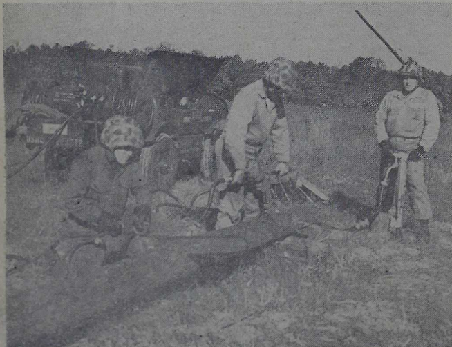
WIRE MEN WORKING —Radio Relay and Const. Co. members begin preparations for setting of a telephone pole. Center man drills hole through which cables will pass after pole is set.
