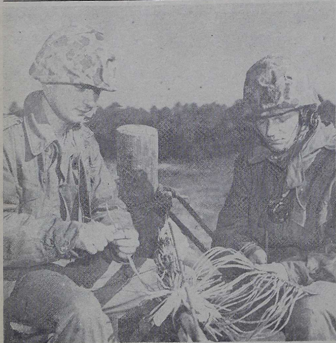
WIRE SPLICERS —Recently trained wiremen splice the lines before connecting circuits. Experienced wiremen are later enrolled at a four-month communication course at Ft. Gordon, Ga.
