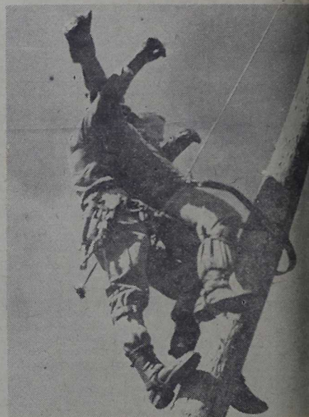
LIFESAVING —All members of Force Troops' 8th Comm. Relay and Const. Co. are indoctrinated in the art of saving "victims" exposed to electric shock. While descending the pole, rescuers are given artificial respiration to the unconscious victims.
