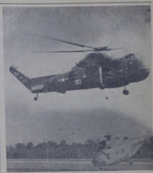
REVERSE RESCUE—This Elizabeth City, N. C., based Coast Guard helicopter gets a 50-mile airlift back to its home from an HMR-461, MCAF. The CG "chopper" crash-landed near Englehart, N. C., losing its tail section when the main rotorblades struck it. MAG-26 was notified and dispatched the "copter to the scene. This sort of operation has become habitual with the squadron, which has made quite a few similar rescue lifts. Moving the "downed" helicopter across land would have required much planning and equipment, many man-hours and tax dollars.
