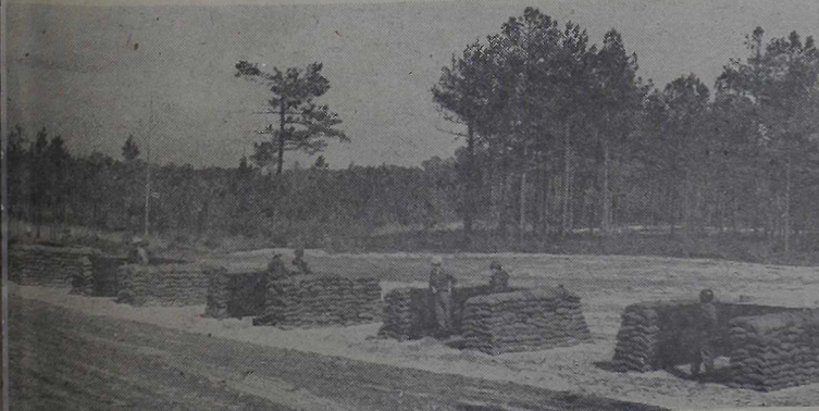
LETHAL PASSES —The F-6 area live-grenade range was officially opened last week by Maj. Gen. P. Riseley, commanding general, MCB. Constructed by members of Bravo Co., 2nd Pioneer Bn., the range will be managed by the Base range office.
