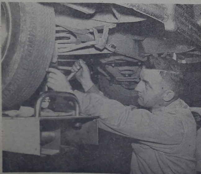
FRONT-END, WHEEL ALIGNMENT —Act. GySgt. Ralph W. Wood, NCOIC of the Automotive Hobby Shop performs about six front-end and wheel alignment jobs daily. This service is done on an appointment basis only.
