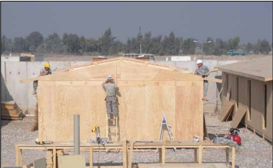
Courtesy photo BAGHDAD — Three Soldiers with 1434th Engineer Company install a roof truss on a building at Contingency Operating Station Deason Jan 16. The standard eight-room building, called a b-hut, will hold 32 additional personnel when complete.
