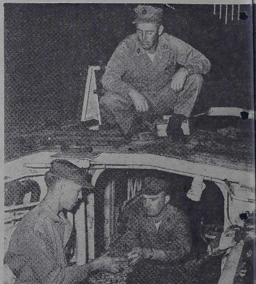
CARBURETOR INSTALLATION —A reconditioned carburetor this is ready for installation on the 810-horsepower Amtrac engine handed to Lance Cpl. J. P. Aylesworth, left, by Act. SSgt. J. Hayden. Act. MSgt. O. V. Peters, battalion maintenance chief, looks on.
