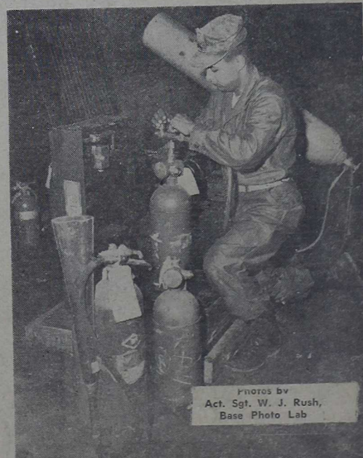
FIRE PREVENTION —Fire extinguishers, four of which are carried in each amphibious vehicle, are re-charged by Cpl. J. Martinez, H&S Co. This service is a part of each maintenance check.
