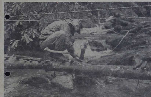
CROSS OVER THE BRIDGE —Marines improvise a bridge across one of the many mountain streams in the area. They use materials at hand to build a walkway and rig handlines for safety measures. Most Marines agree that this type of bridge is superior to treading a tight-rope over streams. (Photo by Act. Sgt. R. D. Crabtree)
