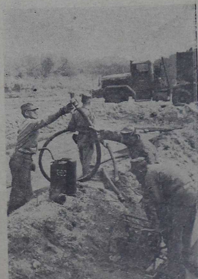
GASOLINE DUMP —Members of the Bulk Fuel Co., Force Troops, fill two of the rubber tanks used for field storage. The company supplied fuel for all Division and Force Troops vehicles during the LANTPHIBEX 1-60 exercise.
