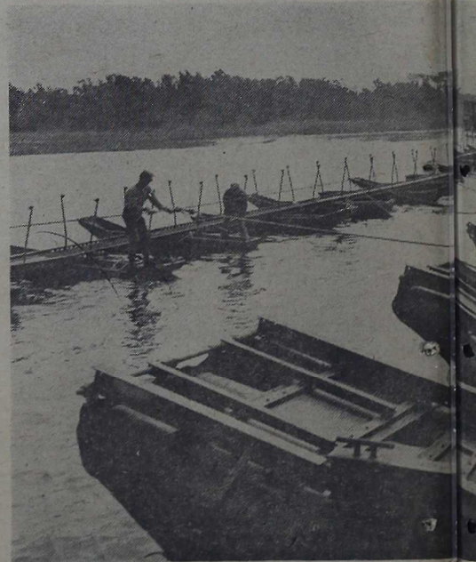
COMBAT BRIDGE —Shortly after friendly forces invaded Onslow Beach, the 8th Engineer Bn., Force Troops, bridged the inland waterway with the pontoon bridge above. The D-Day operation
