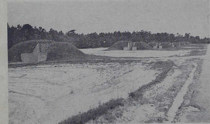
SINGLE IGLOOS —The single earth-covered magazines are made with concrete walls 12 inches thick and have about a foot of dirt over the concrete shell. The single magazines have a barricaded front and are about 200 feet apart.
