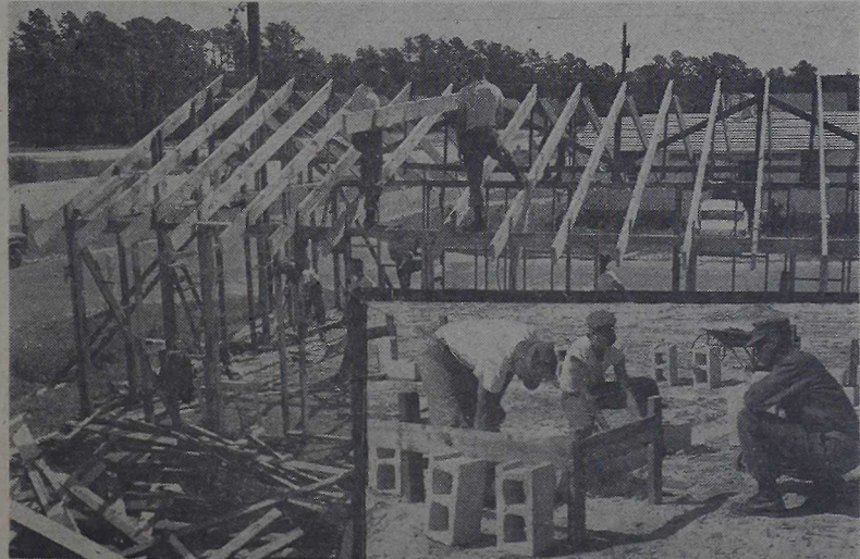
RE-CONSTRUCTION —As Marines of First Infantry Training Regiment (above) tear down a surveyed building at Camp Geiger, after ITR personnel (inset) lay a foundation of cement blocks upon which the lumber from the razed building will be transformed into a new "Combat Town." Three members of the 8th Engineer Bn., Force Troops, are supervising the work. (Photo by Pfc T. J. Mikalajunas)
