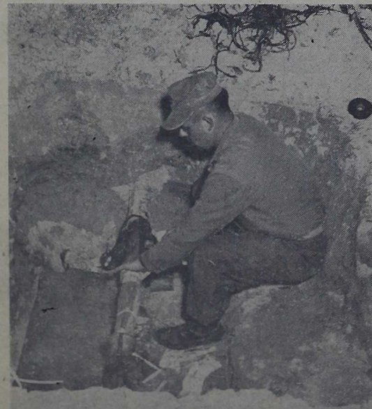
CABLE SPLICING —One of the main trunk lines in the Camp Lejeune area is readied for splicing SSGT. V. A. Gray is but one of the many skilled technicians in the Base telephone section. (Photo by LCpl. G. H. McIntyre)
