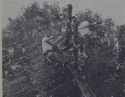
WORKING HIGH —Hundreds of feet of open line must be replaced yearly by telephone repairmen such as Pfc's A. Clifford and T. McGinn. Spiked boots and sturdy safety belts are the marks of these men's trade. (Photo by LCpl. G. H. McIntyre)
