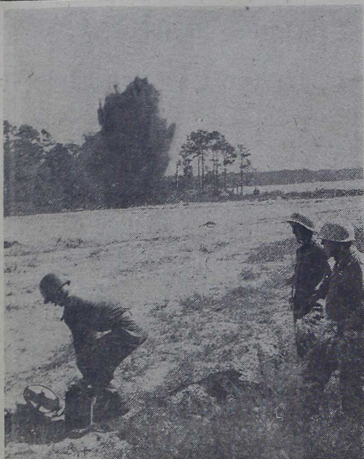
UP SHE GOES—Pfc William R. Keeten, a student at the Demolitions School, pushes the plunger setting off a ditching charge on the Courthouse Bay Demolitions Range. Two demolitions instructors, SSgt. Raymond D. Borque and SSgt. Edward E. D. Carroll, stand by to see that all safety precautions are carried out during the operation. (Photo by SSgt. R. H. Strader)
