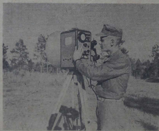
ELECTRONIC CANNON COCKER —SSgt. Richard G. Udell, Hq. Btry., Tenth Marines, operates a tellurometer, a distance-measuring machine, during an artillery firing exercise at Ft. Bragg, N. C. This machine is capable of calculating great distances within a matter of minutes. (Photo by Sgt. Lewis M. Kuritz)
