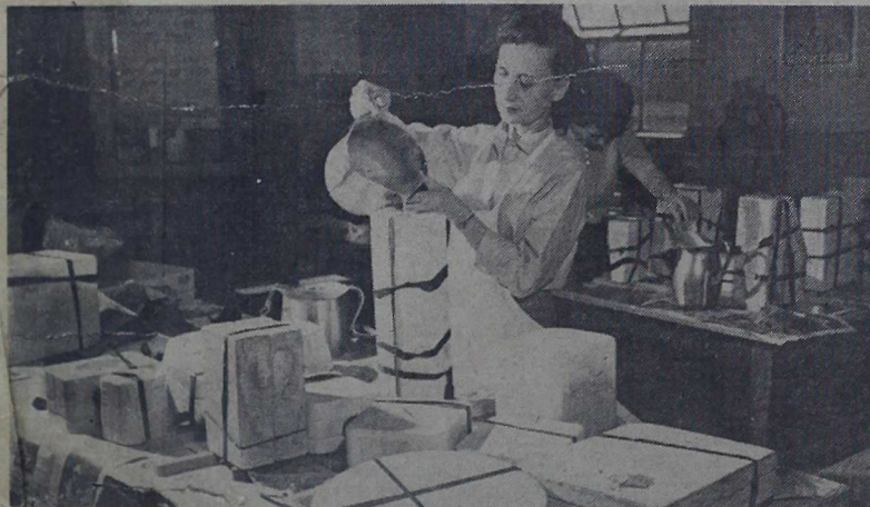
THE BEGINNING—Mrs. Dorothy Byrd pours the ceramics mixture into a mold held together by strips of rubber. The mixture is composed of Tennessee and Kentucky clay, California feldspar and chemical compound. This is the first step in ceramics.
