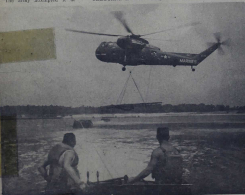
TUG OF WAR — Bridge boats from 2nd Bridge Company battle hurricane-force winds and each other as they attempt to stabilize a pontoon float while the helicopter prepares to lower a section of raft into place on the weaving target. (Photo by GySgt. John Babyack Jr.)
