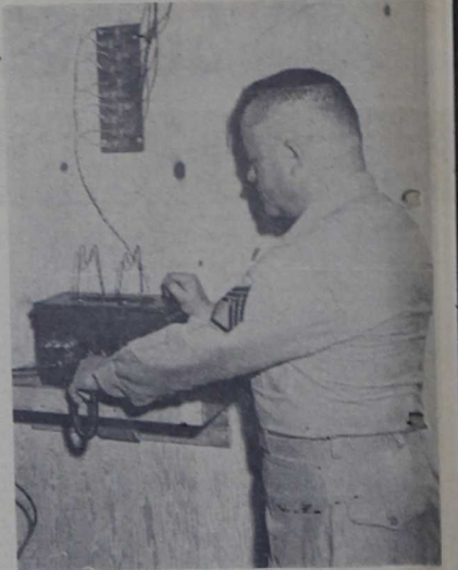
SSGT. WALTER F. KEEFE checks the jacks on the modified switchboard. This second board has several new features but still retains the simplicity of operation as in the first.
