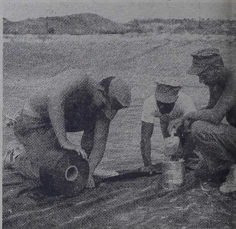
THE KEY TO SUCCESS —And that's an understatement. Co., 8th Engr. Bn., Marines are seen "sealing" the six-inch between the strips of plastic in the basin of Riendeau. These seals, which will require approximately two days must be flawless. Any leak would mean seepage under basin, which eventually would literally uproot the entire
