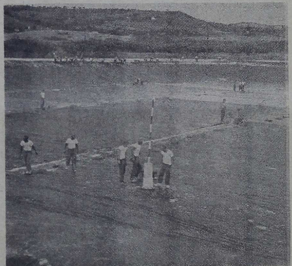
THE FINAL HOURS of construction find numerous operations being carried out on small scale. In the background, Marines put the finishing touches on the five-foot wide strip of sand which covers the entire edge of the reservoir. Here and there, along the seams joining the seven strips of plastic, two and three-man teams make final check on the sealed joints. In the foreground, the drainage standpipe, through which the reservoir will get its water supply, is given a last-minute check. The job is almost over.
