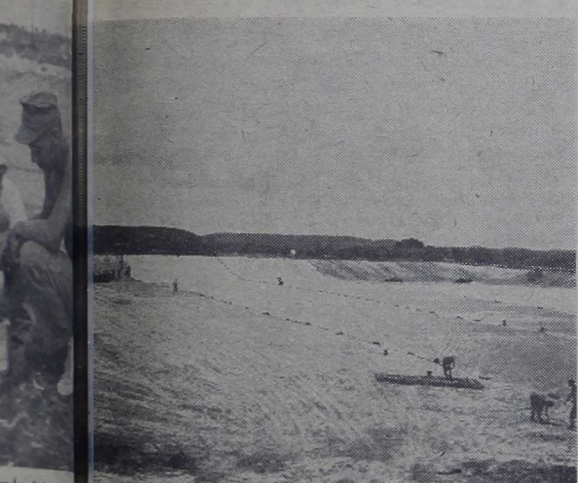
DOWN, THREE TO GO —With construction well under way, four of seven strips of polyvinyl chloride are seen in the left, at the far side of the reservoir, the plastic, in rolls, finally comes, awaits placement in the basin of the reservoir.
