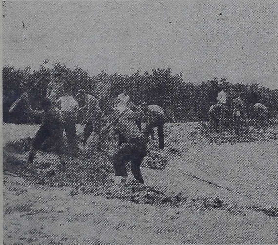
BURIED TREASURE? —No, but the fast and furious pace of those shovels does signify the final phase in the construction of Riendeau Reservoir by the engineers of "D" Co., 8th Engr. Bn. The men are spreading sand around the edge of the reservoir from the top down for approximately five feet in two to four inch layers. This will protect the edge of the vinyl from the sun in case the water level should sharply decrease for any reason.
